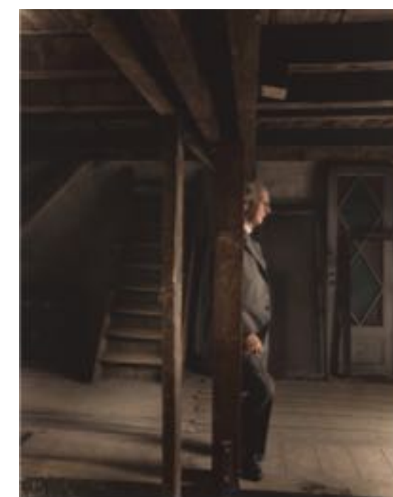
ALL POSTS, BEAMS, AND SUPPORTS ARE ROUGH CUT TIMBER AS SEEN IN REFERENCE IMAGE. BEAMS ARE 4"x6" AND SUPPORTS AND POSTS ARE 4"x4". ALL ARE WORN AT CORNERS.
